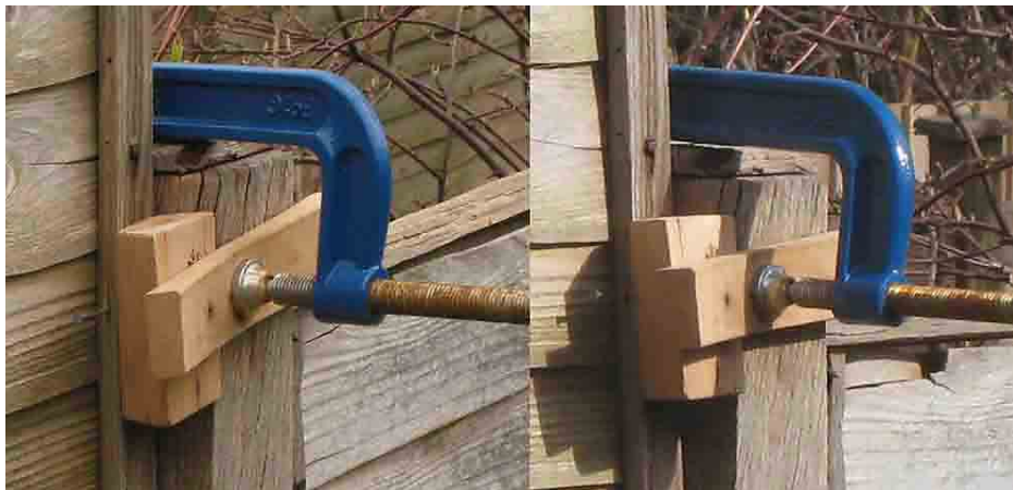
Fig. 12 Fence Repair (1) Overcast sky, (2) Sunlight.
